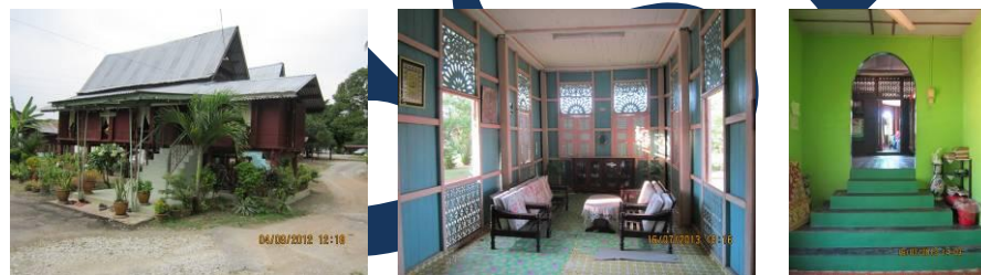
Figure 6: The geometry of high pitched roof, on-stilts structure, quality of materials, surface, craftsmanship and spatial segmentation of frontal and posterior zones contribute to the high level of values in the originality of Malay traditional house design. Photos taken by authors.
